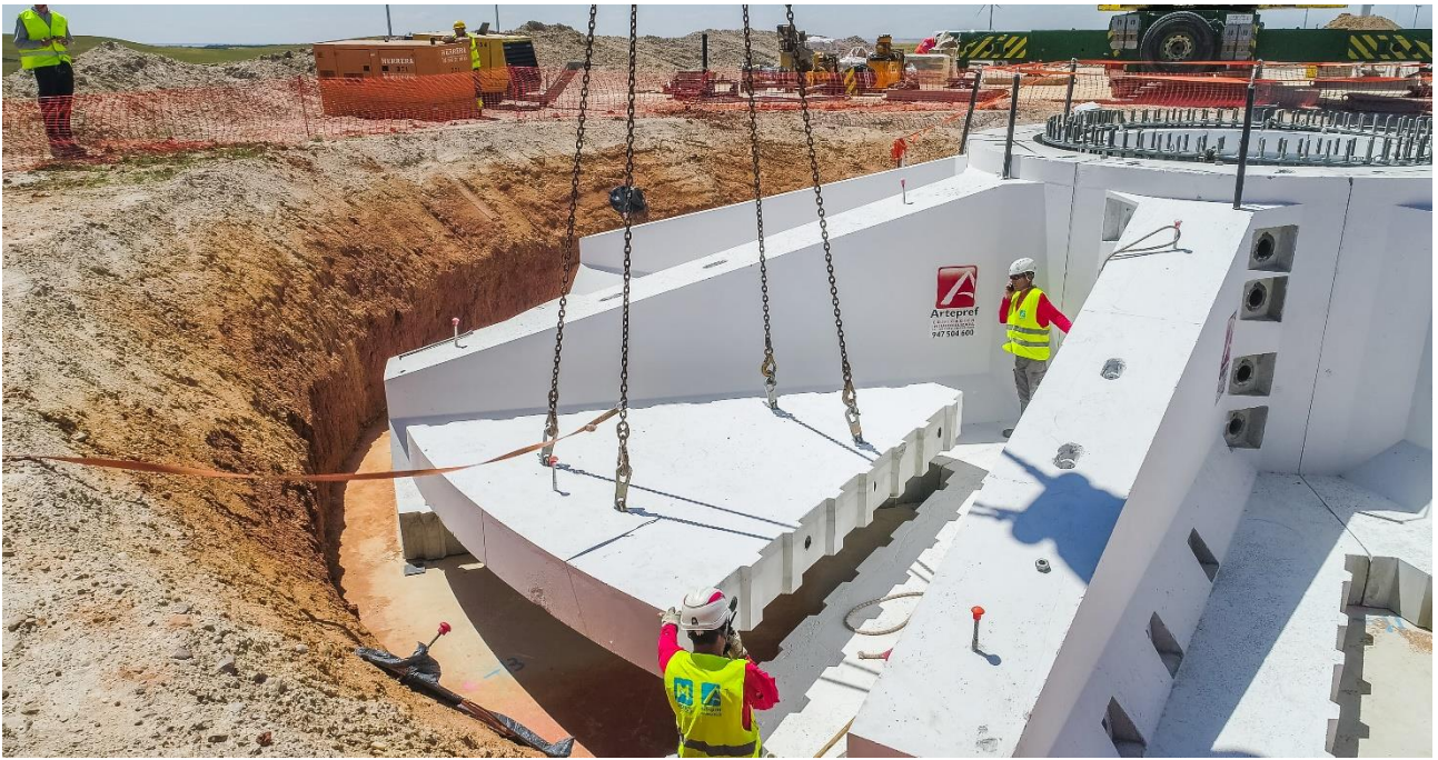
image during the assembly phase of the secondary elements
