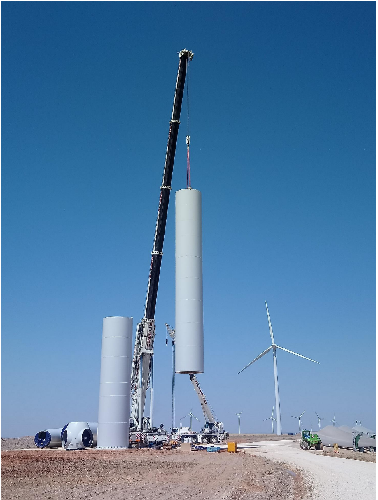
image during the assembly phase of the steel tower
