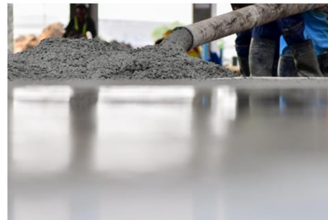
Concrete being poured at a construction site. Image via Shutterstock/Bannafarsai
