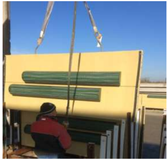
Figure 26. Lifting on site of walls with absorbers Sollevamento in opera pareti con assorbitori
