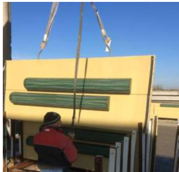
Figure 26. Lifting on site of walls with absorbers Sollevamento in opera pareti con assorbitori
