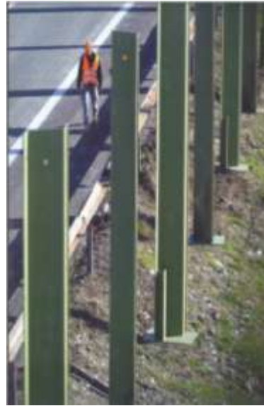
Figure 14. Plates-risers infilled in the ground ready for HC wall slabs installations
