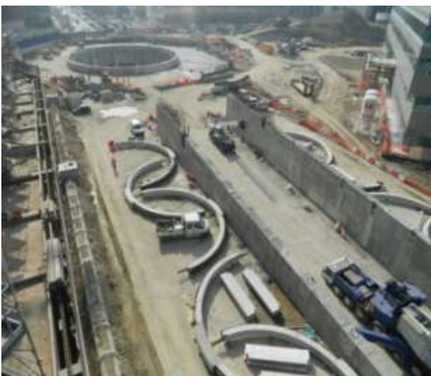
Figure 1. Arches (precast in 3 pieces) assembly in situ Archi (prefabbricati in 3 segmenti) assemblati a terra
