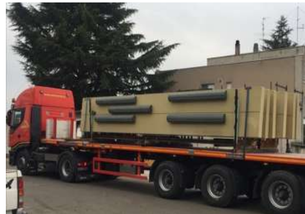
Figure 25. Transport on racks to erection site Trasporto su rastrelliere al cantiere
