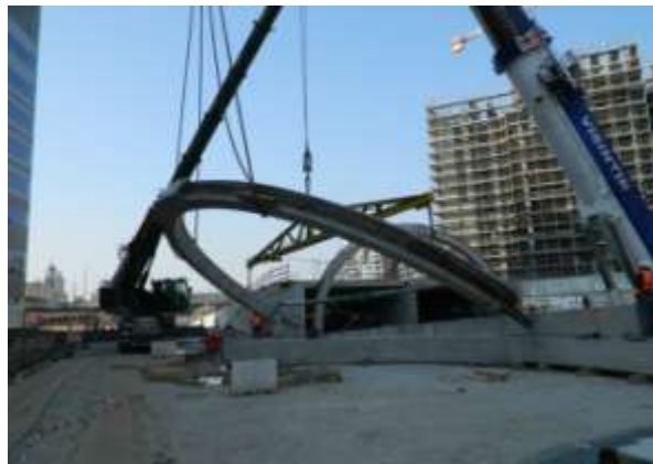
Figure 3. Lifting/tilting of the arch (with 2 mobile cranes) Sollevamento/basculamento arco (con 2 autogru)
