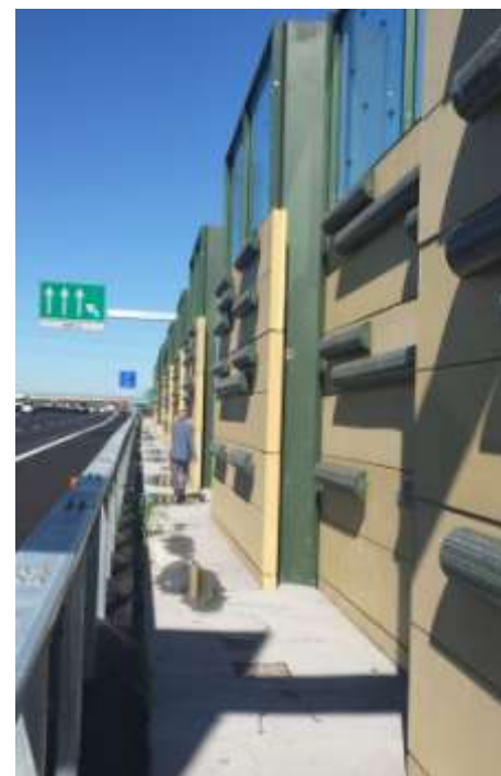
Figure 30. View of installed barrier with upper glass Vista di barriere con vetri superiori
