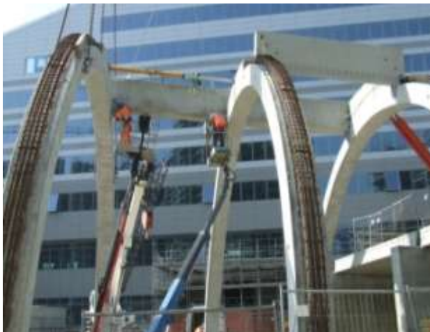
Figure 4. Installation of upper bracing walls Posa velette superiori di irrigidimento
