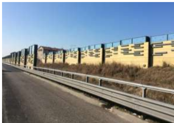
Figure 31. View of installed noise barrier Vista di barriere installate
