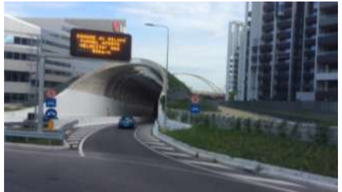
Figure 11. View of tunnel completed Vista del tunnel completato
