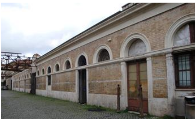
Figura 2. Vista Padiglione 2B/ View Pavilion 2B
