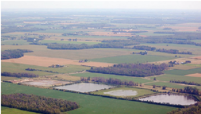
Figure 2. Grand Bend Area Wastewater Treatment Facility, South Huron, Ontario
