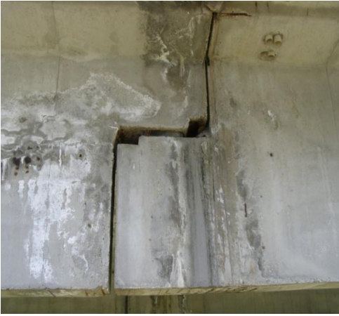
Figure 8: Particular of cantilever girder)/particolare sella gerber.
